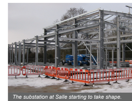
The substation at Salle starting to take shape.
